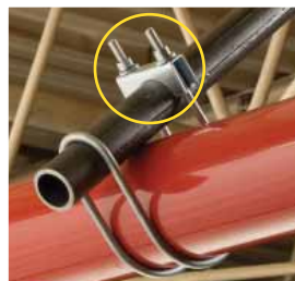
Step 5: Tighten bolts until heads shear off.
